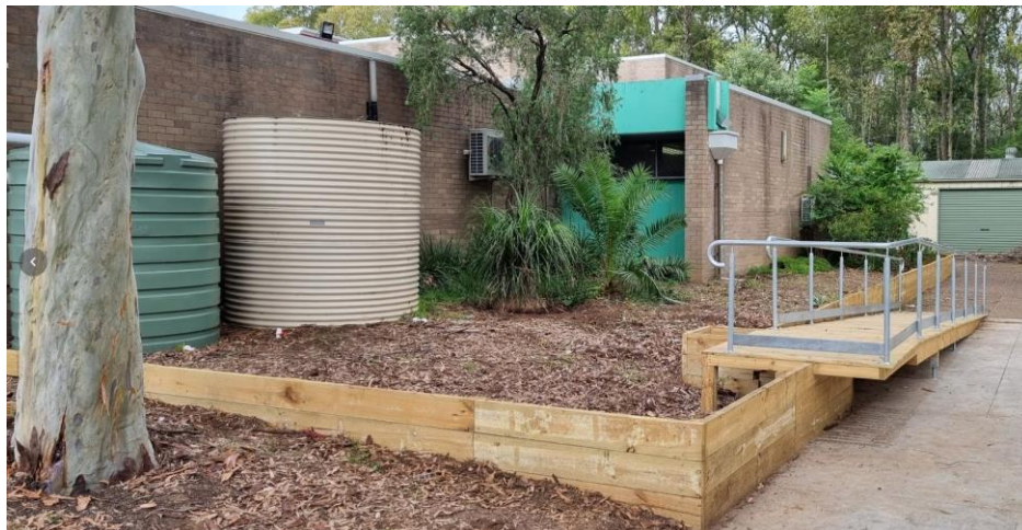
2 - Construction in Progress March 2023
